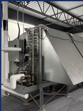
Insulated Drain Pan with Hot Gas Loop & Heat Trace: Enables complete and fast defrost
