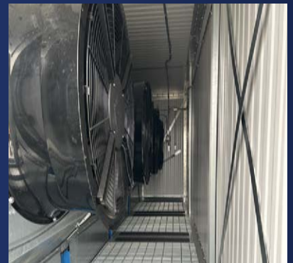
EC Fan Motors in Insulated Penthouse: Precision airflow with built in fan speed control
