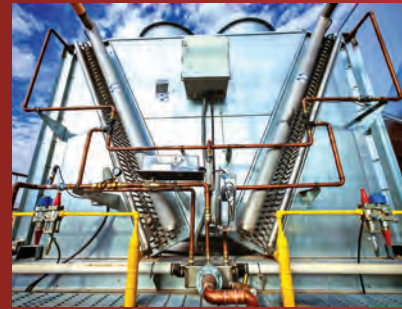
Water Recirculation System: Optimizes water usage while maintaining peak cooling performance.
