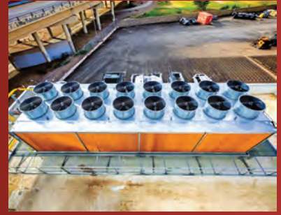
16 Fan V-Bank Design: Provides high-capacity, efficient cooling
