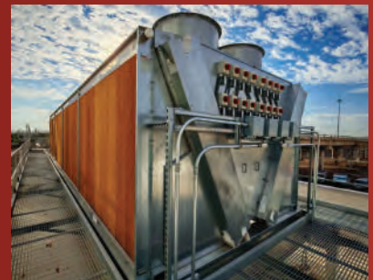
Controls Integration & Adiabatic Pads: Fully integrates with refrigeration system for efficient operation and water management.
