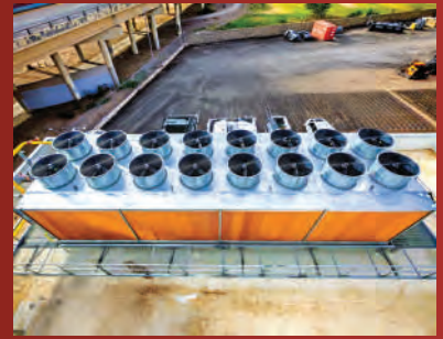
16 Fan V-Bank Design: Provides high-capacity, efficient cooling
