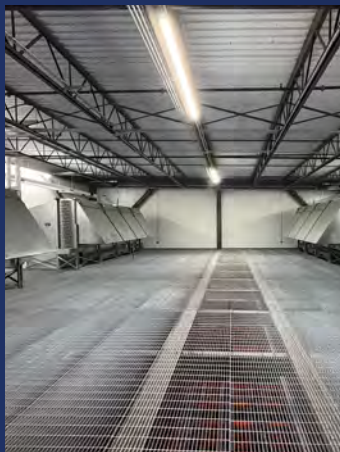
Inlet Air Hood: Provides more effective defrost and directs return airflow
