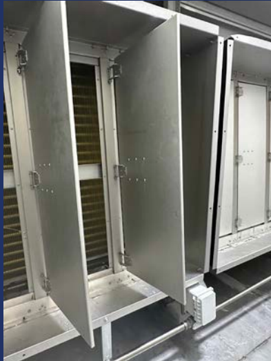
Louvers automatically close during defrost cycle – Epoxy coated fin material
