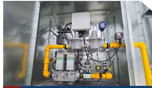
02 Direct Fire Burner Controls
