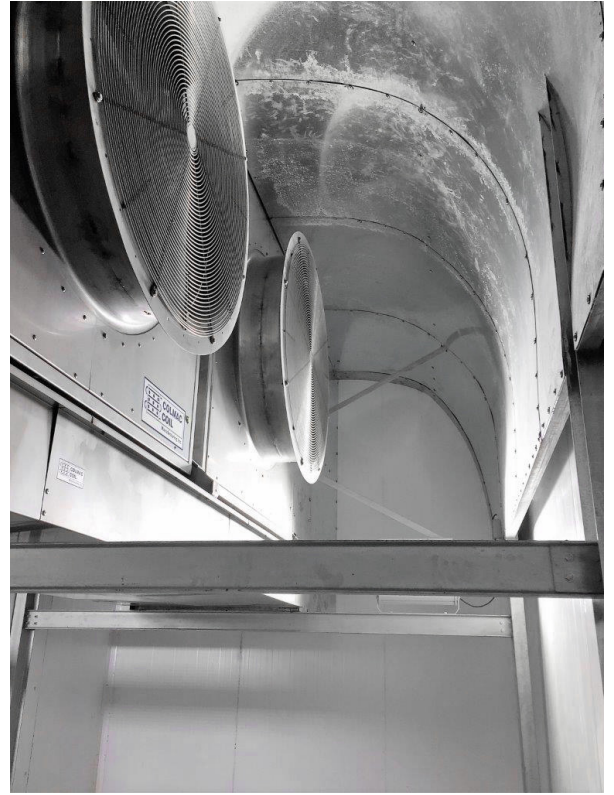
Interior of Blast Cell
