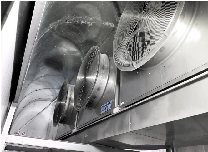
Interior of Blast Cell
