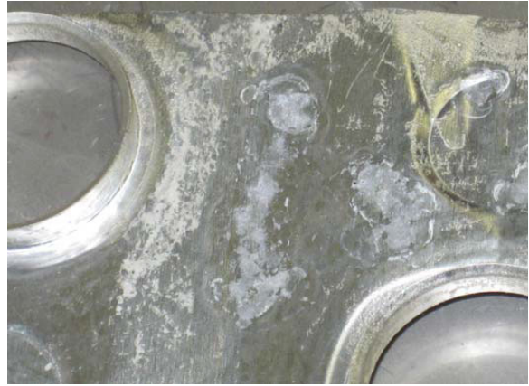
Figure 9: Aluminum 1100 after 250 hours submerged in a .16% Sunny-Sol 150 water solution
