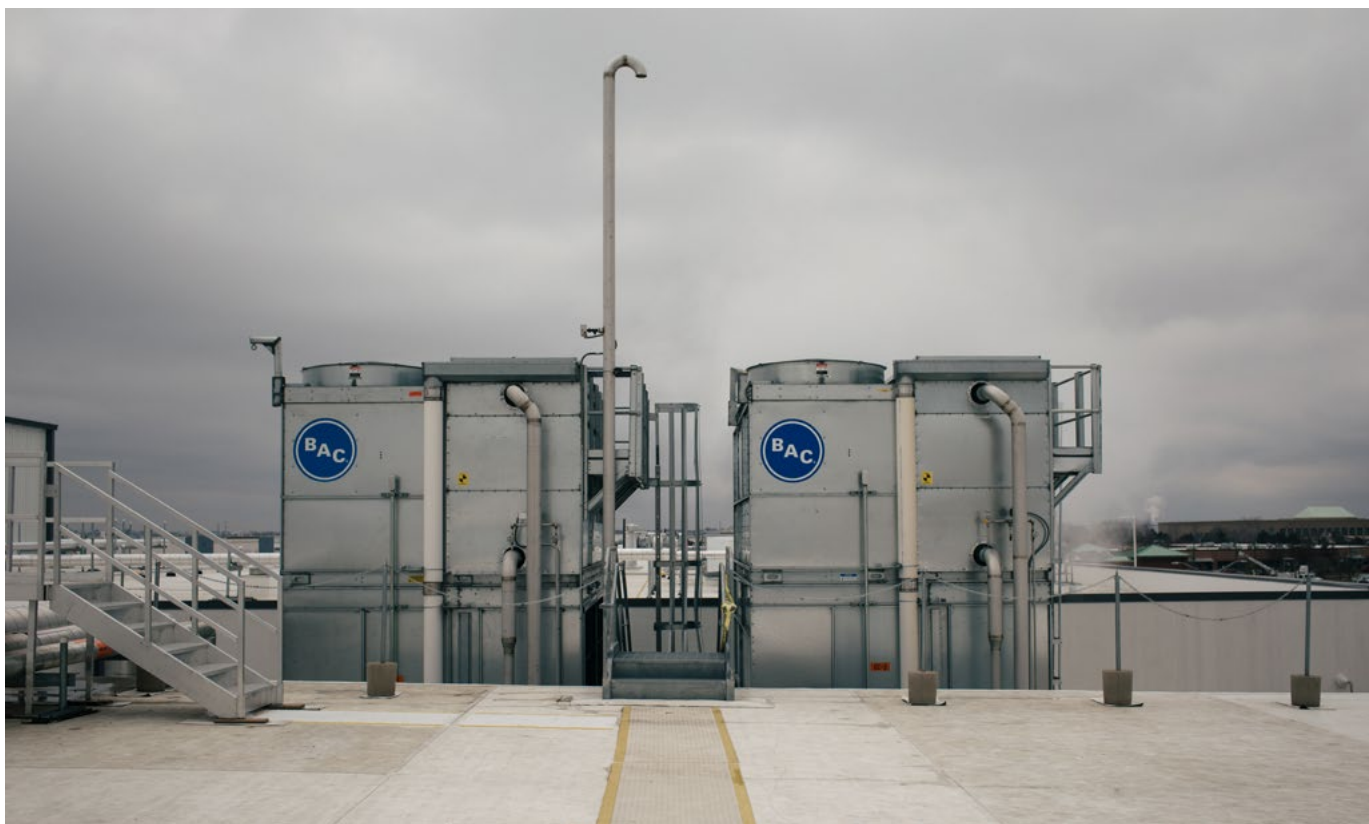
BAC evaporative condensers above the engine room
